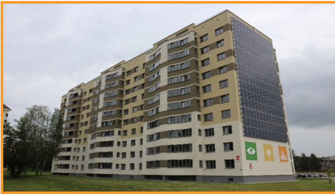
Fig 1. Energy efficient residential building in Hrodna.
